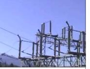
The potential between the two lines is 500kV, that's half a megavolt! At these potentials the air molecules get ionized, becoming plasma, the air becomes a conductor transfering electricity creating an impressive electric discharge. The video was taken in BC Canada.
